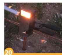
20 Thermowelding has finished
