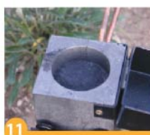
11 Thermoweld powder discharged.
