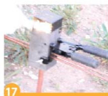
17 Thermoweld powder fired.
