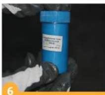
6 Take the thermoweld powder box
