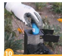
10 Discharge the thermoweld powder into the mould.
