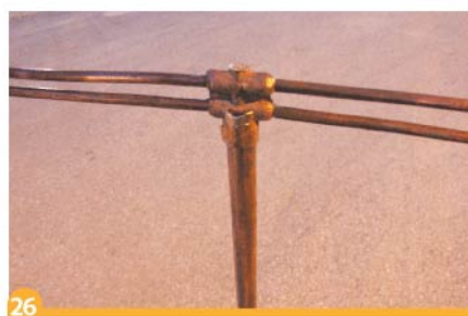
Welded earthing conductors and earthing electro.
