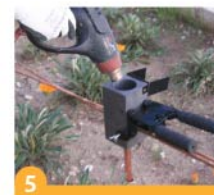
5 To prepare for heating inside of the mould
