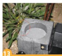
13 Thermoweld system is ready for fire.
